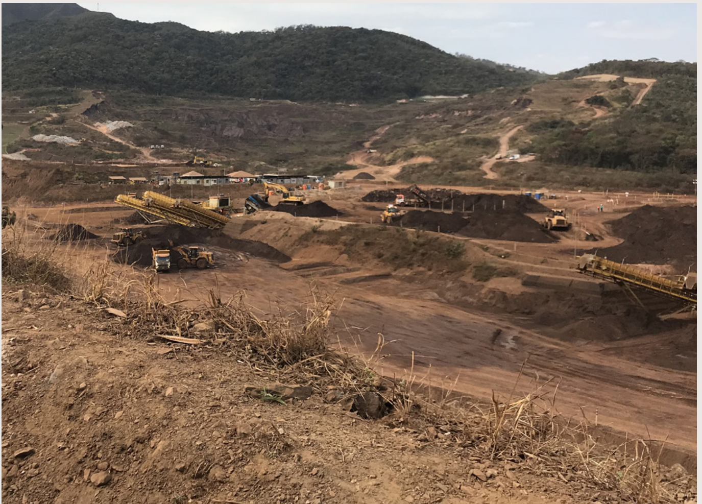
The collapsed tailings dam at Brumadino and the excavations taking place to find the four remaining bodies
